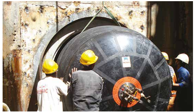
Pronal pipeline stoppers can be deployed quickly and easily to provide environmental protection and maintenance worker safety
