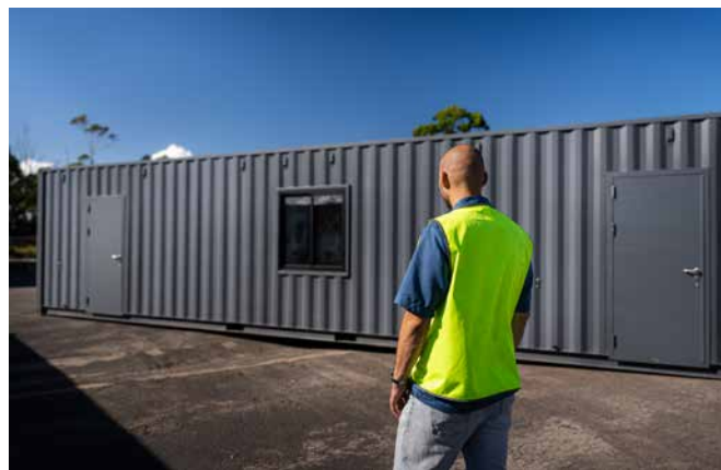
A 12 m x 2.4 m Express Office featuring a separate restroom under construction at Modulate's Mayfield facility.
