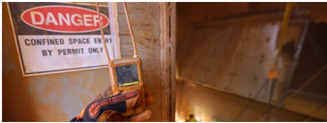
Confined spaces can present maintenance hazards and delays to production resuming after breakdowns
