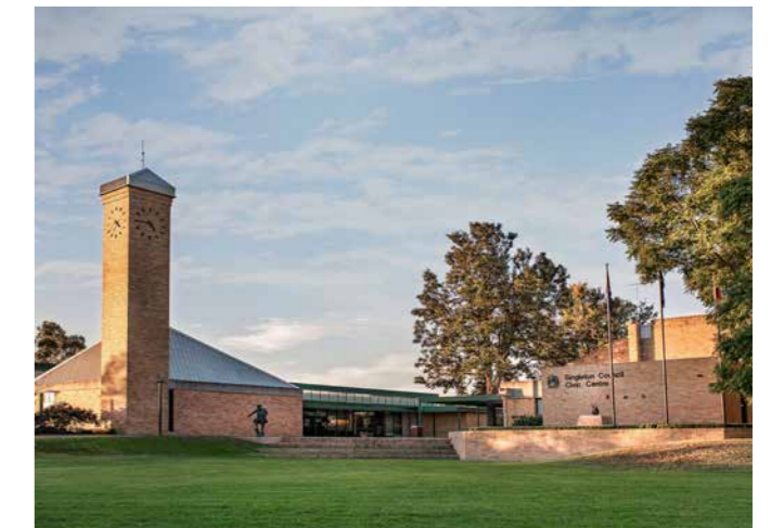
Singleton Council Administration Building
